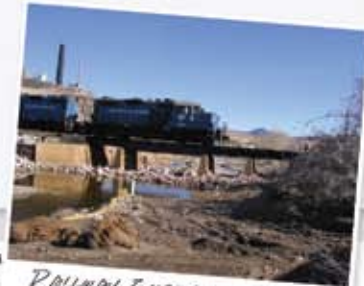
RAILROAD EMERGENCY REPAIR
