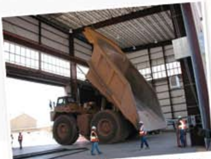
CARLOTA MINE TRUCK SHOP
