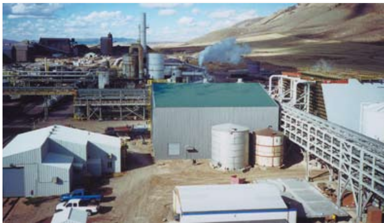
Jacobs Engineering, Phosphate Processing Plant, Conda, ID
